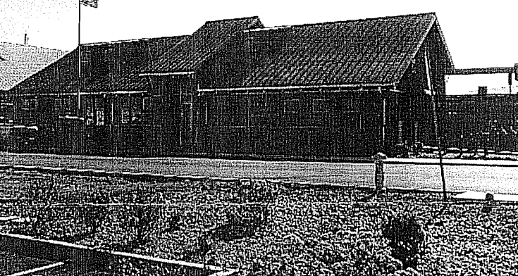
Waste Water Treatment Plant
